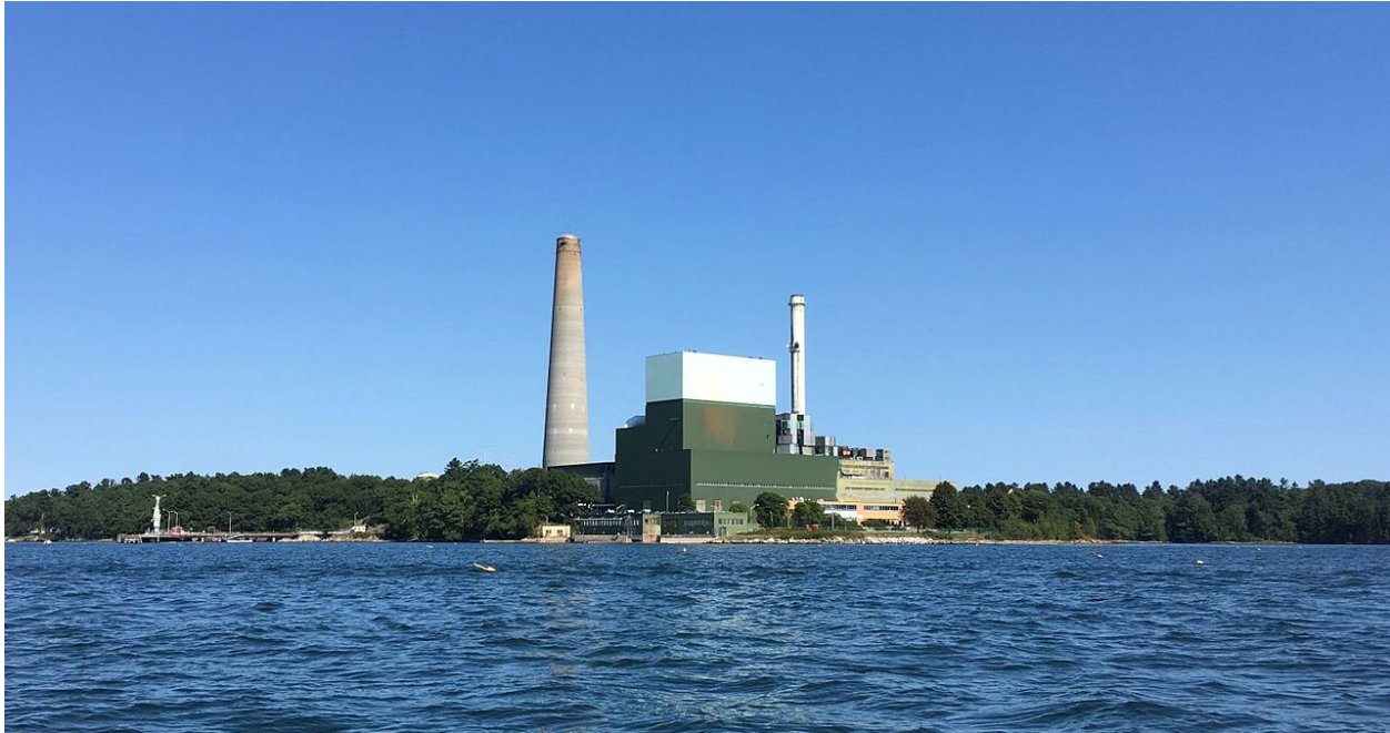
Figure 8: Oil-Fired Generation Plant. Wyman Station in Yarmouth, Maine is an 810 megawatt oil-fired generation plant. This plant was originally built in 1957-58 and has been updated several times with Unit 4, its largest unit, beginning operation in 1978. Pollution controls were installed in the early 2000s. EMP protection for pollution controls needs engineering study. Photo credit: Wikimedia Commons/NewTestLeper79
