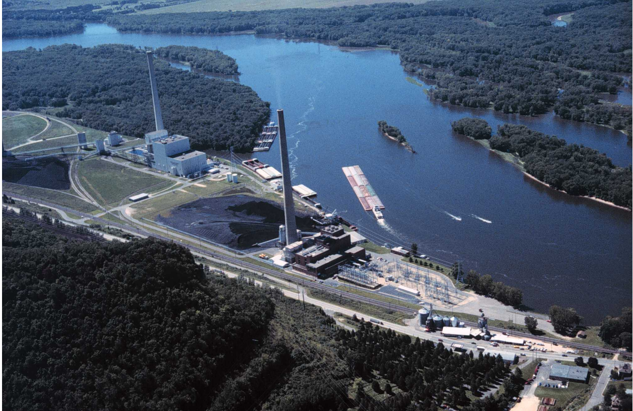
Figure 7: Coal-Fired Generation Plant Complex. The John P. Madgett Station (left) and Alma Station (center, now decommissioned) in Wisconsin are coal-fired generation plants. The EMP vulnerability of coal-fired plants with complex fuel handling systems from the coal pile (center) to the furnaces near the smokestacks needs engineering study. Photo credit: Wikipedia/USGS .
