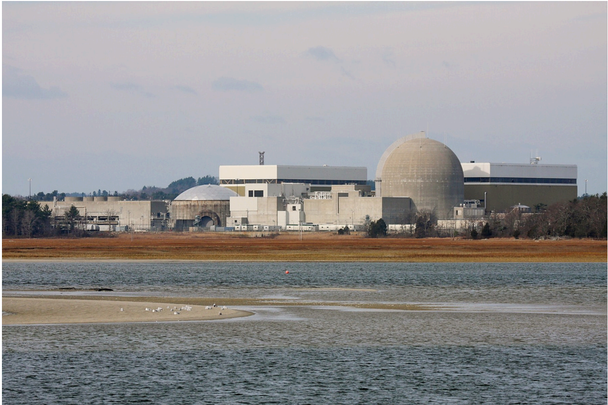
Figure 9: Nuclear Power Plant. Seabrook Station, New Hampshire is in a region susceptible to GIC during solar storms. The plant's 1,244 megawatt output requires use of single-phase GSUs. During a November 10, 1998 solar storm, vibrations induced by GIC caused a four-inch bolt to shake loose in the Phase "A" transformer. Subsequent melting caused loss of the transformer and several weeks of downtime. Photo credit: Creative Commons/Jim Richmond
